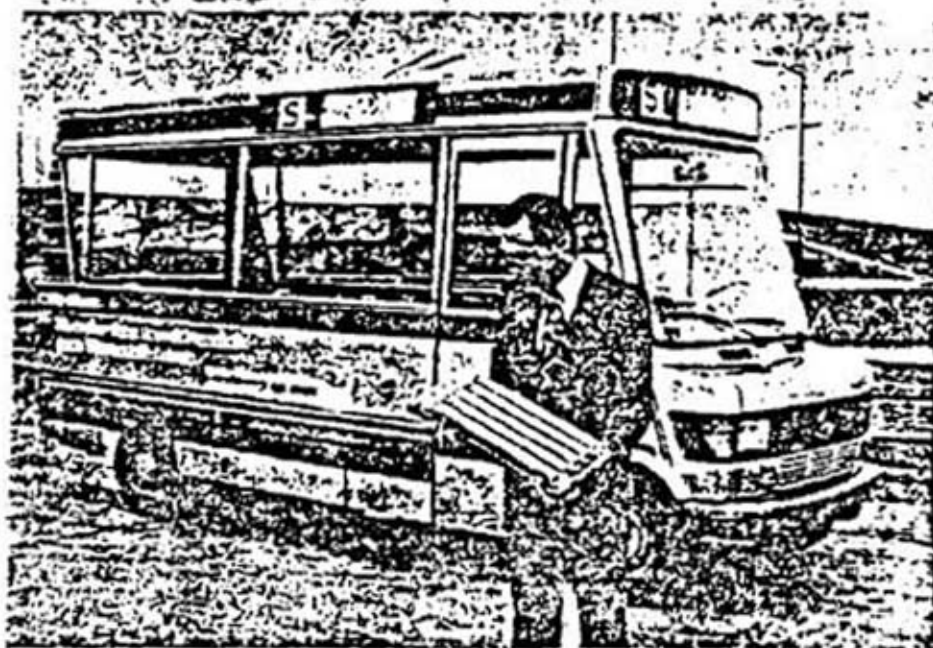
Dr. Helmut Buchner, Mercedes' hydrogen-project leader, displays model of hydride container that replaces gas tank on jitney behind him. Hydrogen-absorb-
